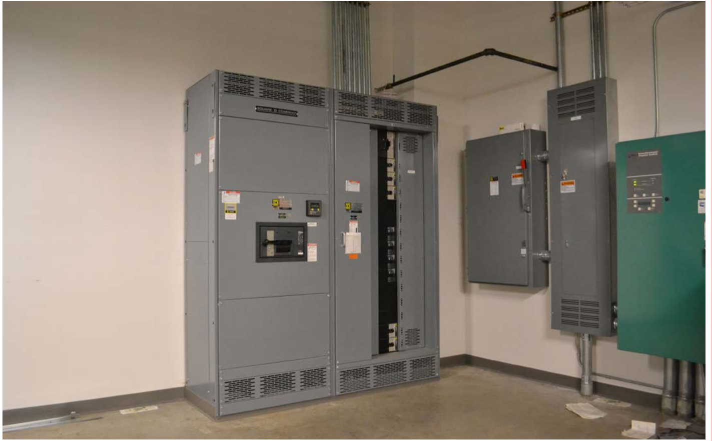
ELECTRICAL SERVICE PANELS, 120/208 VOLTS, 3 PHASE
