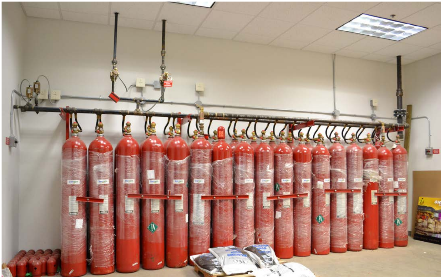
DRY FIRE EXTINGUISHER SYSTEM FOR DATA CENTER
